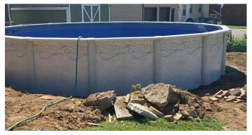
Some jobs have a little rock in the ground when we dig, so be aware that your yard could have the same. It is important for the bottom of the pool base around the outside to have dirt pushed up around it to help contain the sand.
